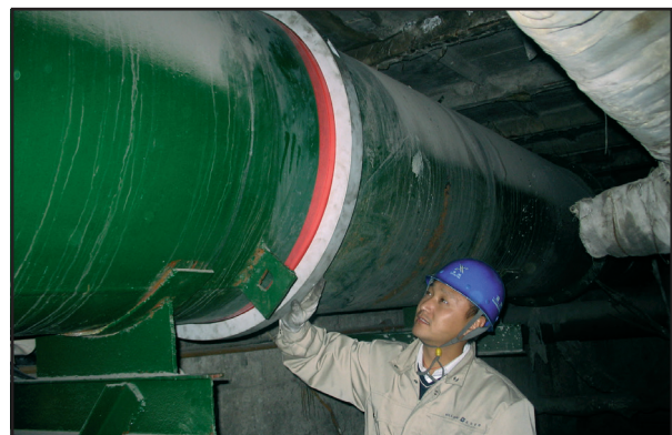
40" Ring on a feed pipe in China (steel industry)
