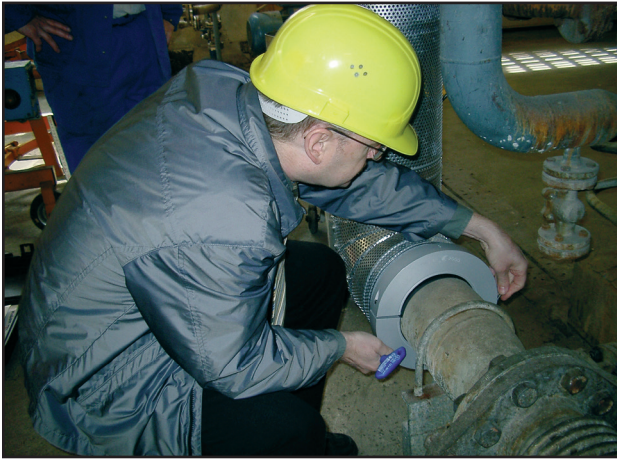
Installation of a 8" Ring at an industrial facility
